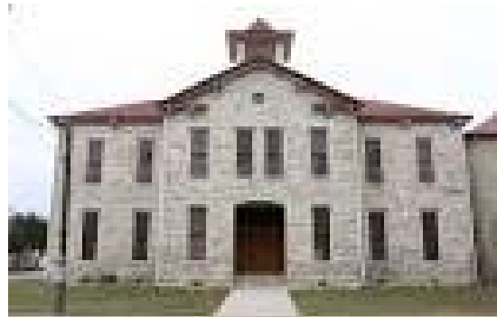
The Navarro building originally opened in 1886 as an elementary school. Today is serves as an academy for grades 9 th through 12 th .
